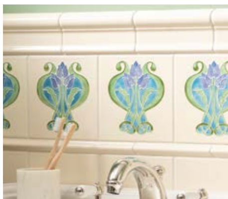
▲ Tiles and mouldings can be aligned, or offset relative to each other. Here, staggered mouldings create a less regimented look.
